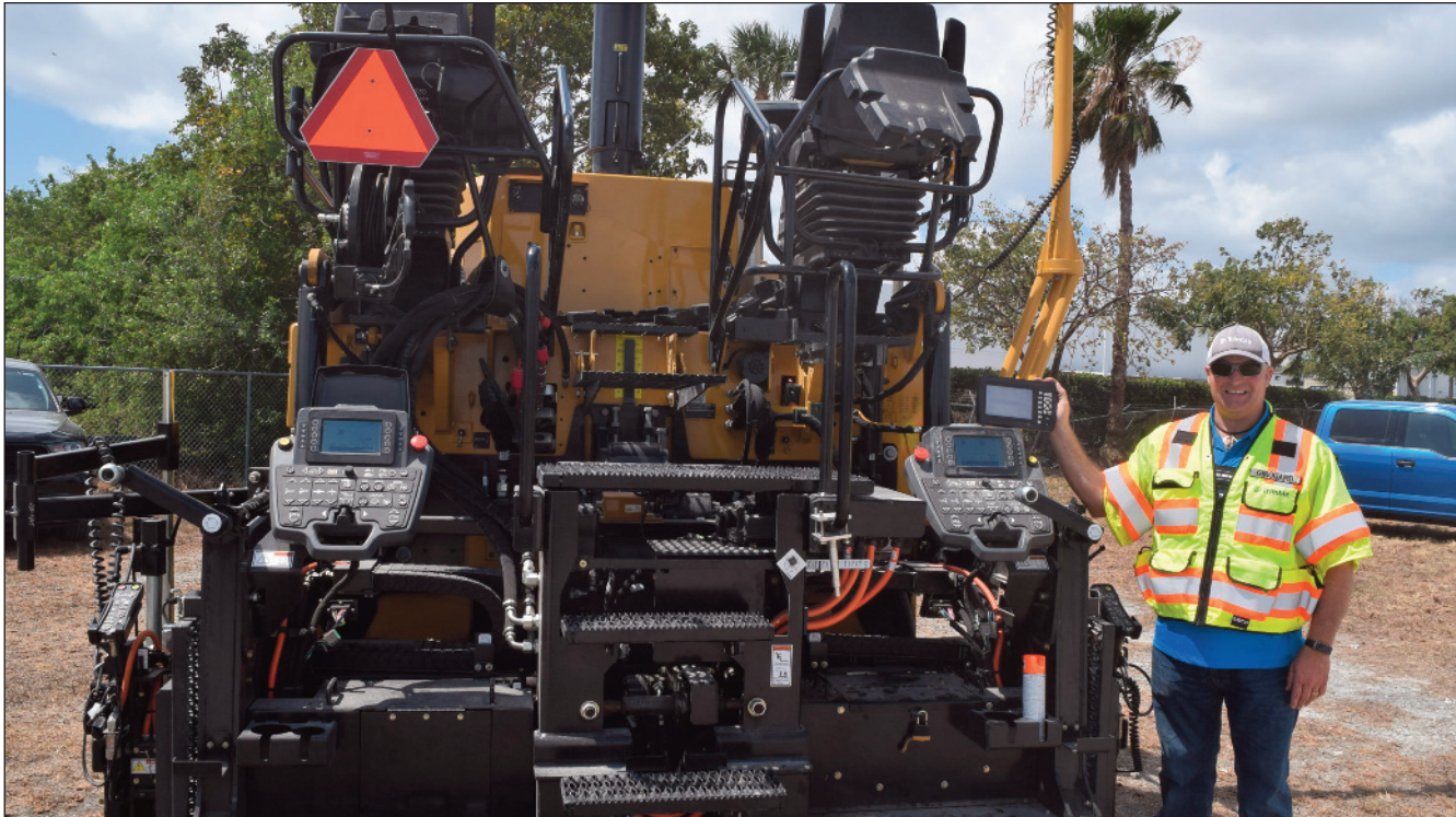
Brian Girouard, SITECH sales/application engineer from North Las Vegas, spoke with contractors about this Caterpillar AP 500 paver and the Trimble Paving Control System that helps speed up paving production while laying a smoother surface and reducing material costs.
